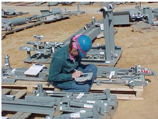
FIG. 3: Worker receiving pipe support using RFID (Jaselskis et al. 2003)
