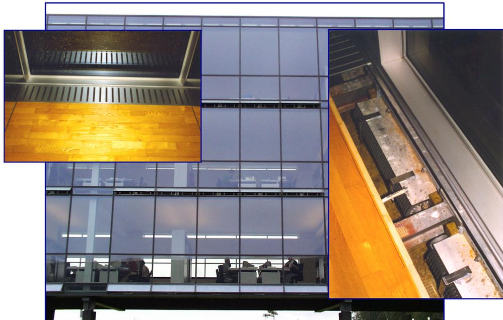
*FIG. 24: Top: B&O Headquarter, Denmark. Bottom: Close up of inlet openings.*
