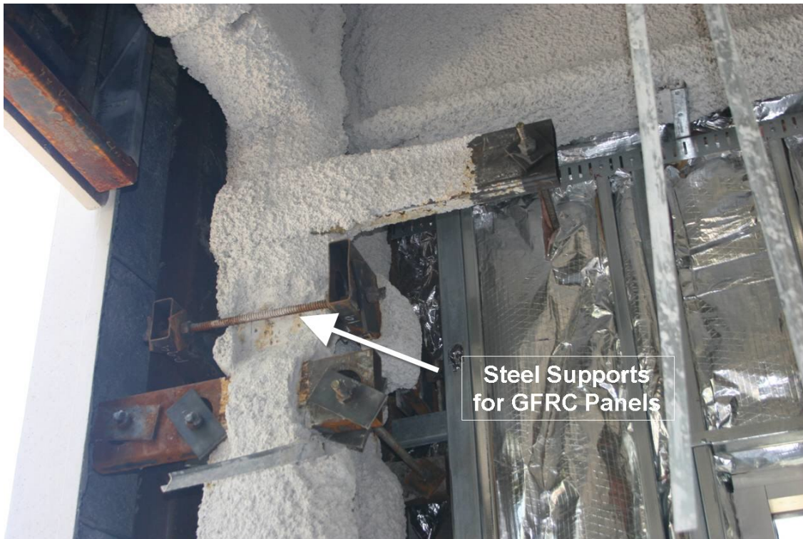
FIG. 12: Figure shows the miscellaneous steel supports for the GFRC panels. The virtual 3D model of the supports was not created which resulted in conflicts with Rain water leaders (plumbing drains) in a couple of locations.
