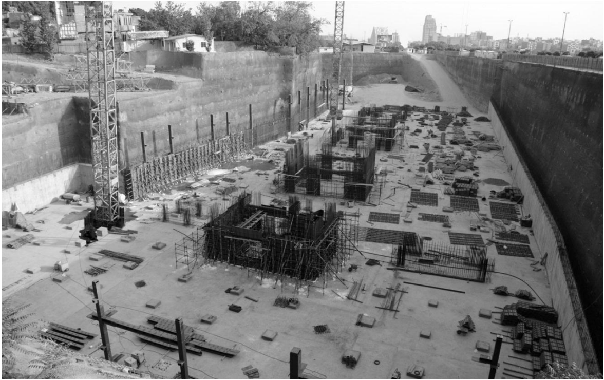
FIG. 9: General view of the case study project under construction
