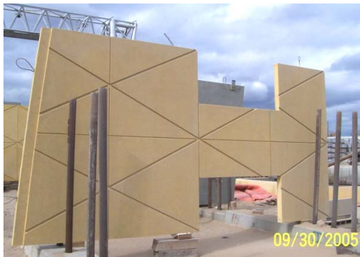
Fig. 5 – Blackfoot Crossing – completed piece in the precast yard.
