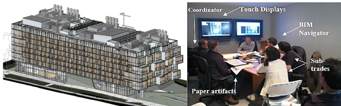
FIG. 3: Integrated BIM model of the UBC Pharmaceutical Building (left) (image courtesy of Hughes Condon Marler Architects) and BIM Trailer used during design coordination on site (right).
