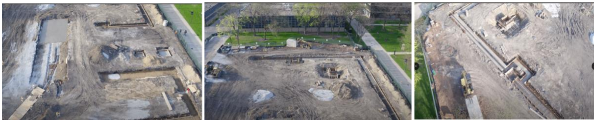
FIG. 1: UAV Dynamic visualization of construction processes and resources from a construction site.
